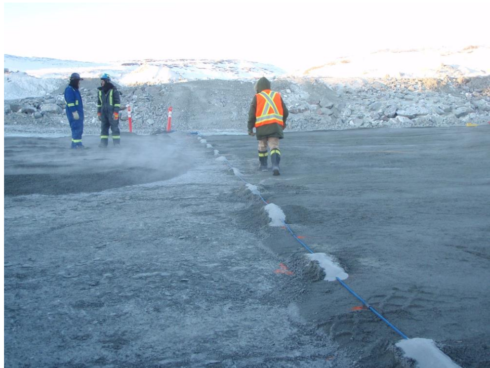
Photo 6: Thermistor cable was graded within the accuracy of the DGPS (20mm). Bentonite water stops were poured between beads. View looking to the downstream side.
