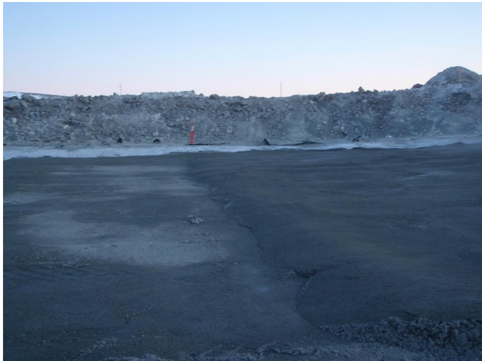
Photo 7: Thermistor cable buried with a slight speed bump of protective FCM cover. View looking to the upstream side.
