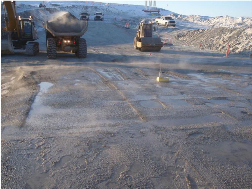
Photo 4: The first several truck loads were slightly over-wetted; water was bleeding out in into thin puddles. All material passed density testing.
