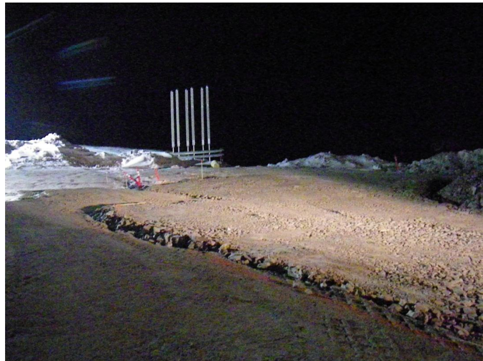
Photo 9: Transition and ROQ material placed from approximately station 1+55 to 0+40.
