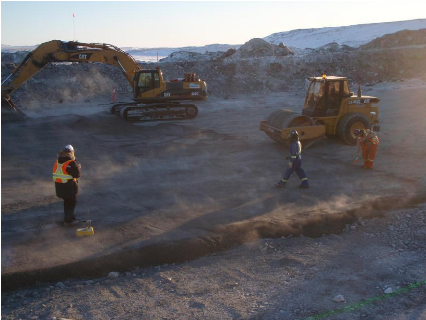
Photo 5: Material as it became drier toward the center of the key-trench. Minimum saturation recorded at 84% after compaction.
