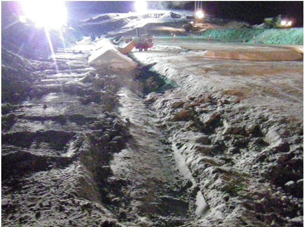
Photo 10: Looking south west along trench at exposed HDPE liner and hoarding over liner. Photo taken from around station 1+60.
